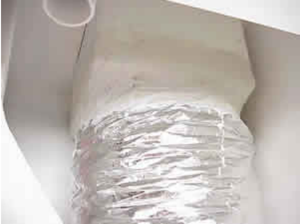
Figure 4. Example of good mastic return connection seal.
