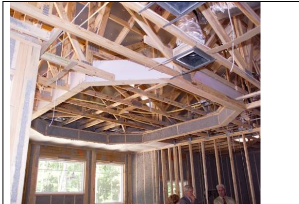
Figure 3 Solid blocking at tray ceiling framing (GWR).
